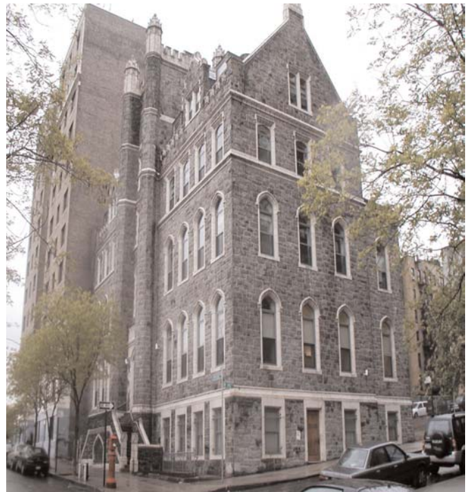
The Fortune Academy opened in 2002 to provide emergency and longer-term housing for 59 ex-prisoners.
